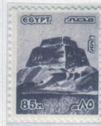
Maidum Step Pyramid. Two of its steps have collapsed.
